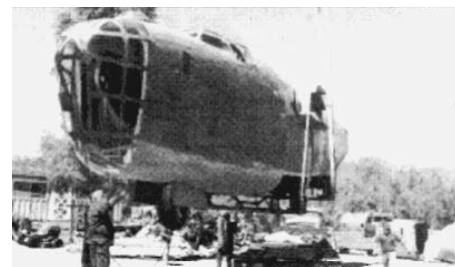
Crane lifting the 7,200-pound B-24 fuselage onto the waiting flatbed.
