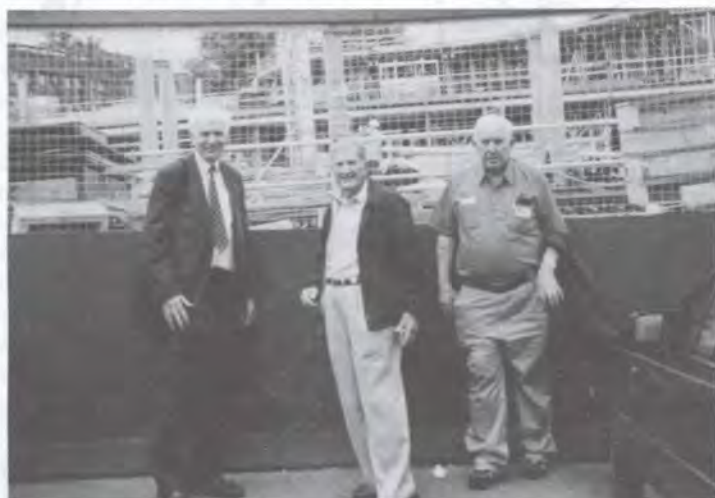
Hilary Hammond, Lew Lyle and Harry Gobrecht at 2AD Memorial Library construction site. (Walt Brown took the picture.)
